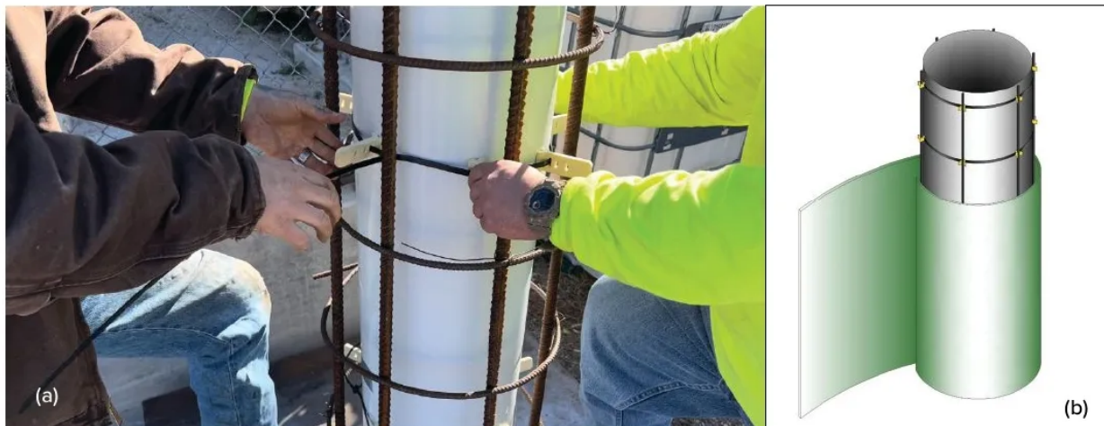
Fig 2: Spacers being installed (a) and the FLF laminate being wrapped around a deteriorated column (b)
